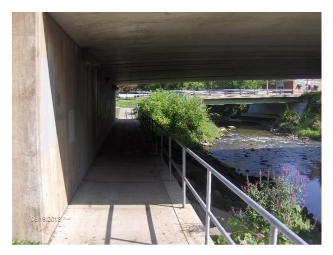
Permits would be required from NYSDOT, NYSDEC, and USACOE. Construction would include the placement of large stones under the highways at the creek's edge along the eastern most wall of the two box tunnels and placing a concrete slab on top forming the trail. Amendities would include LED solar lighting, safety railing, signage, and trail connections including contour earth moving, filter fabric, crushed limestone (crusher run/runner crush), and stone dust for about 800 linear feet of trail.
